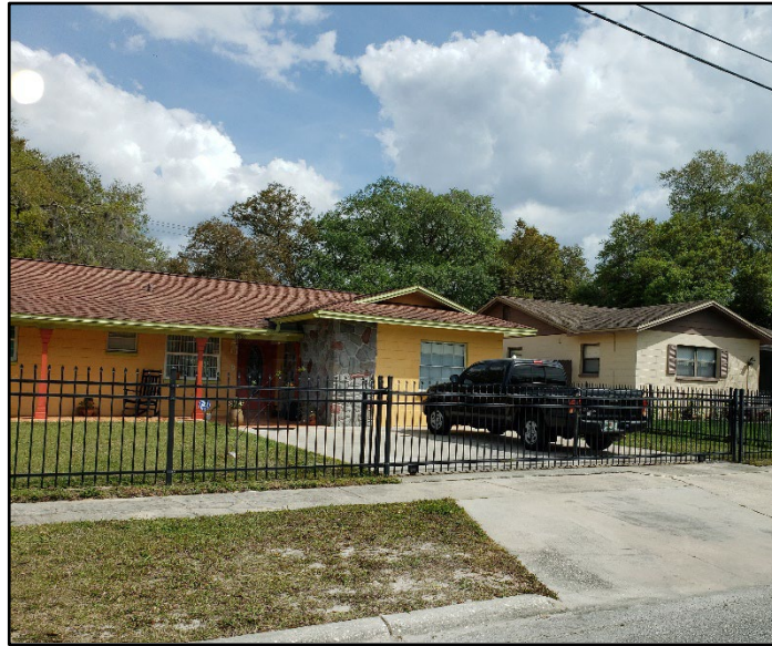
Typical homes in Temple Park
