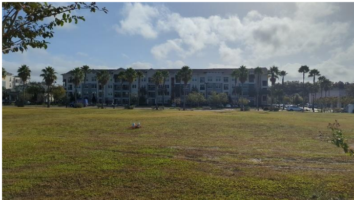
Easterly View of Subject
